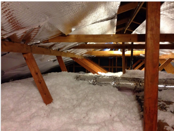
Attic framing and insulation from access hatch
