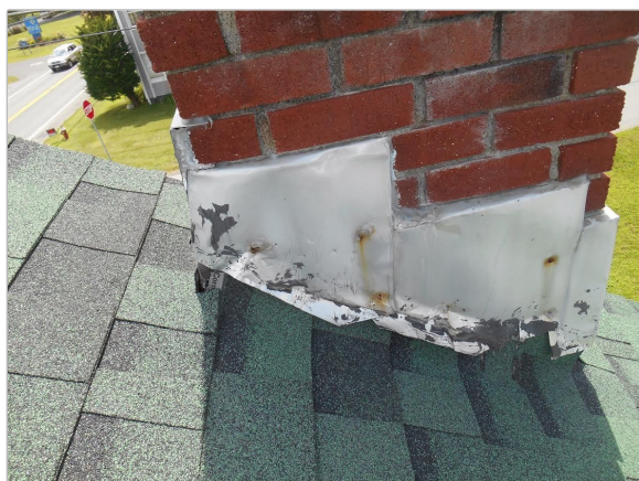
Chimney base flashing, uphill side
