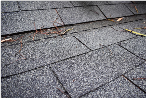
Main roof plane, viewed from ladder at eave
