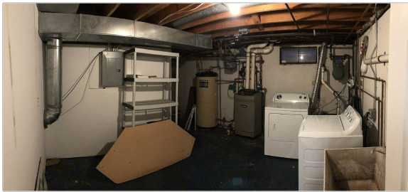
Unfinished basement, mechanical side
