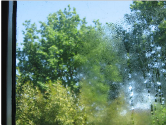
Interpane condensation, living-room window
